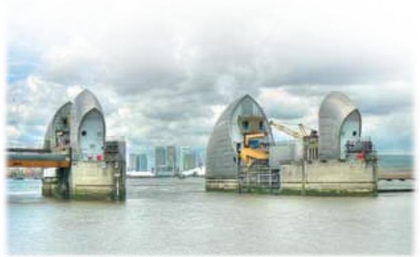
The Thames Barrier at Woolwich is a series of gates which protect London against extremely high tides
